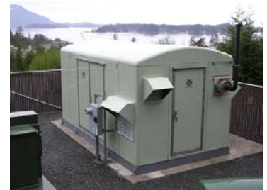
Shown Above: FRP Enclosure for housing high voltage circuits
